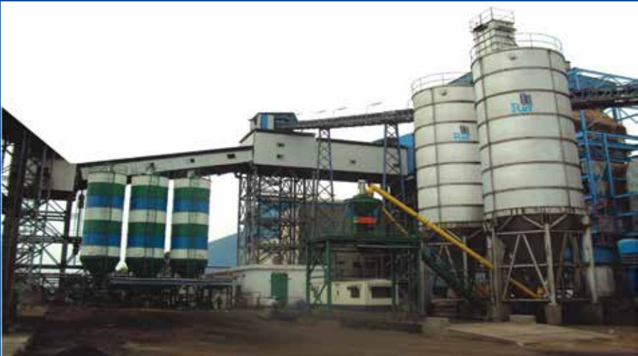
Fly Ash Improvement Plant
